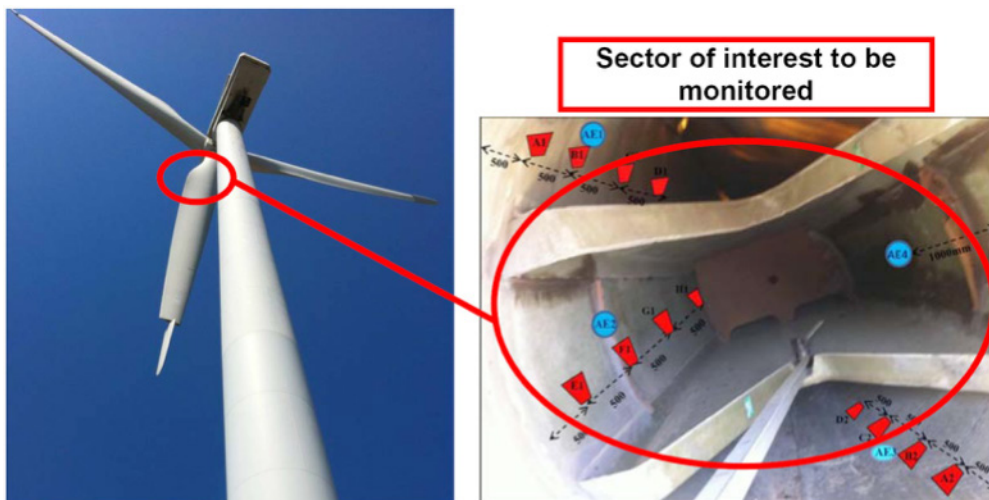
The sector of interest and the internal structure of the wind turbine blade to be monitored, positions of transducers
