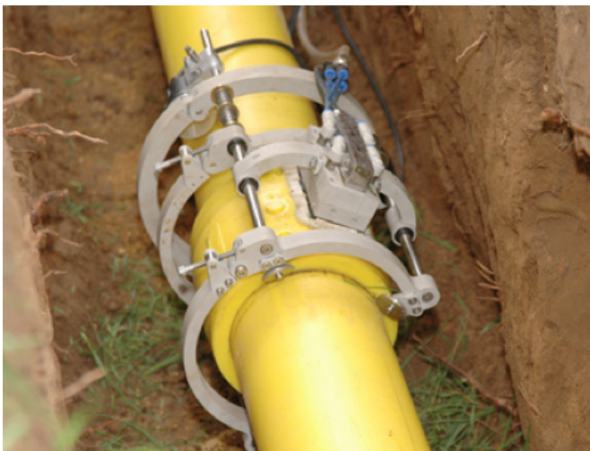
Example of ultrasonic testing of the welded plastic pipe
